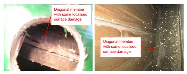
Figure 9: View through inspection hole at top of Panel 8 and a view down into Panel 8
