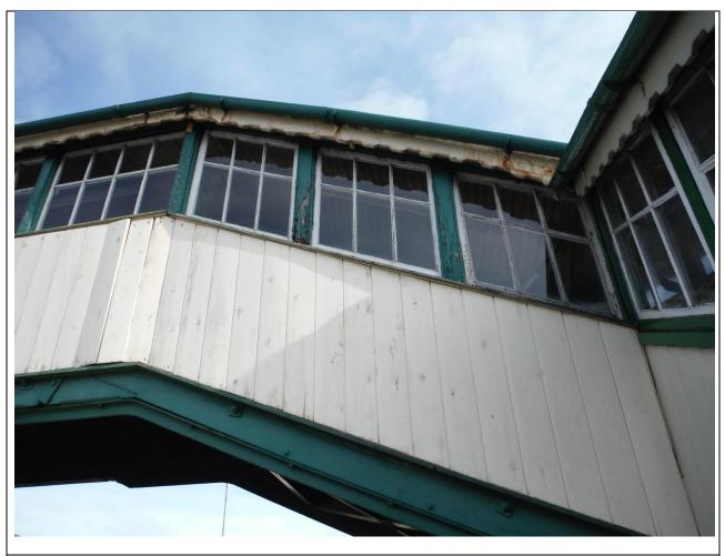
Photo 10: leaking gutter allowing water to spill onto country end face of the footbridge causing paint to peel and degrade timbers (Platform 2)
