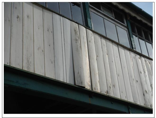
Photo 11: Swelling of timber cladding caused by rainfall. Cladding requires refixing to ensure it does not become dislodged in high winds (Platform 1)
