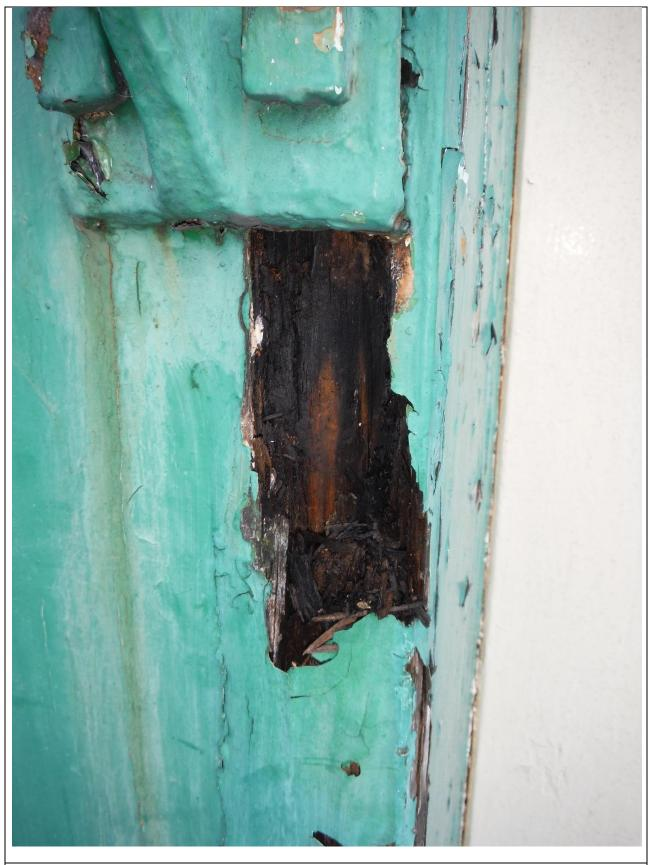
Photo 8: Wet rot of timber at steel T-section connection at westernmost corner directly below roof leak (Platform 2)
