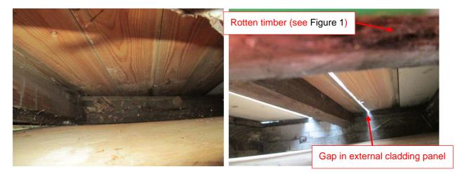
Figure 4: View down into Panel 1 and view down into Panel 2
