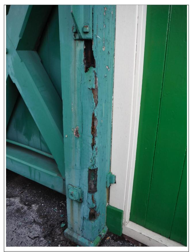
Photo 9: Wet rot of timber at steel T-section connection at westernmost corner directly below roof leak (Platform 2)
