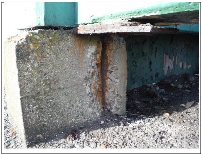
Photo 4: Minor spalling and corrosion of reinforcement at southernmost of 4 post column concrete base support (Platform 1)
