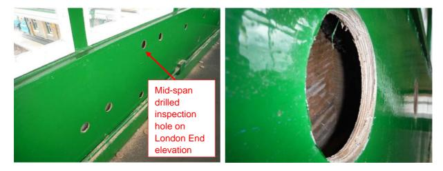
Figure 2: Drilled inspection hole showing diagonal member transition into horizontal member
