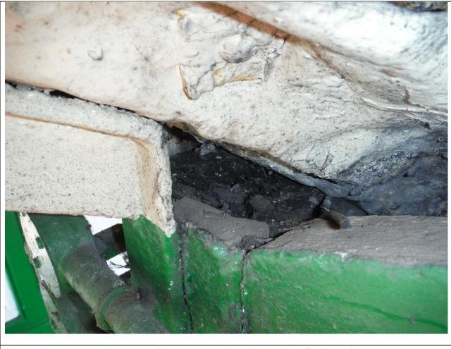
Photo 7: Wet rot to top of vertical roof support timber directly below leak (Platform 2)
