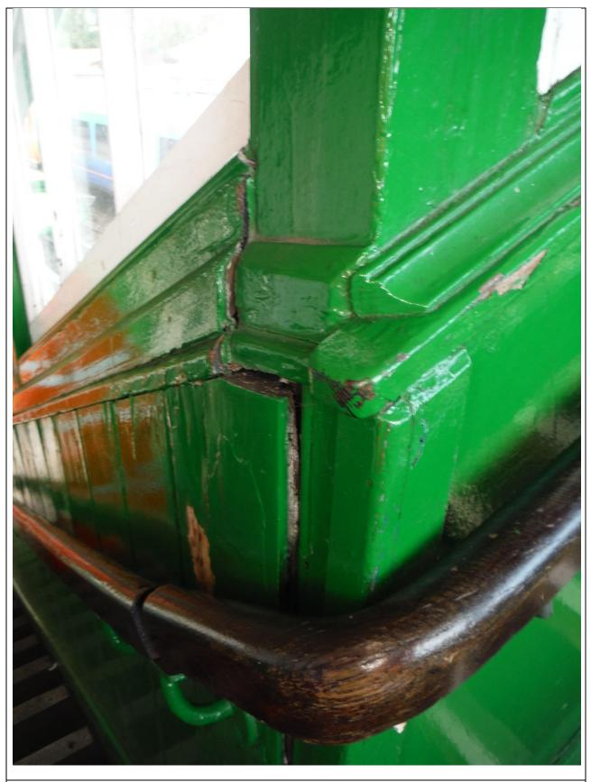
Photo 6: Roof leak above causing swelling and separation of stair corner joint (Platform 2)
