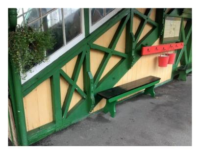
Figure 4 – Alton station footbridge stair elevation on platform 3 showing original bracing.
