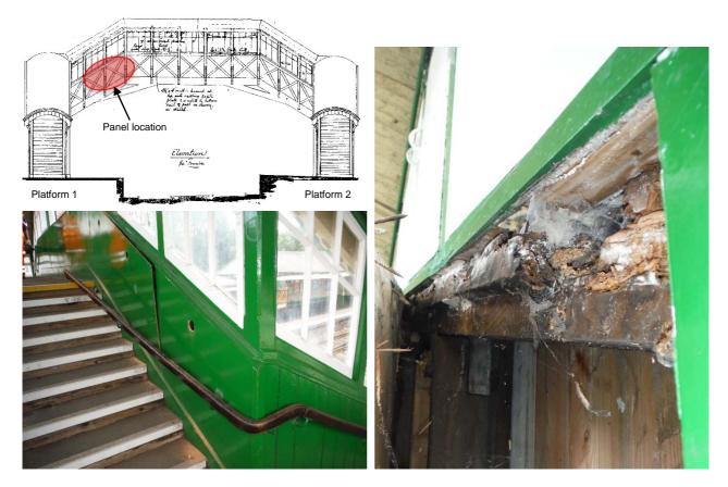
Figure 1: Location and rotten timber behind internal panel
