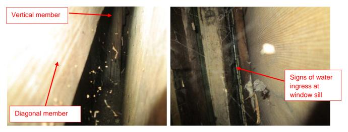
Figure 7: View towards Platform 1 and a view looking up to the window sill in Panel 5
