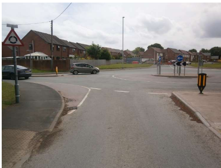
Photograph 4: Lack of deflection prior to roundabout
