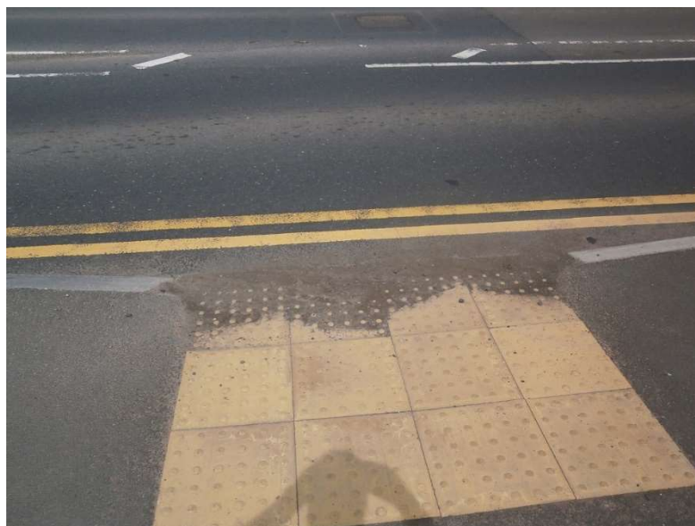
Photograph 5: Build-up of detritus material at crossing point on A458 east of roundabout
