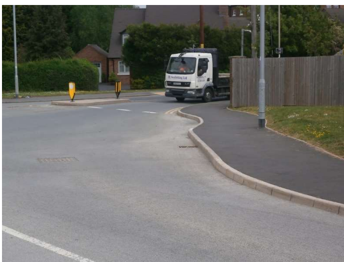
Photograph 5: Build up of detritus material on circulatory carriageway
