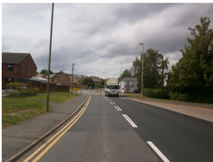
Photograph 3: Lack of deflection on approach (Westbound) to roundabout towards Shrewsbury
