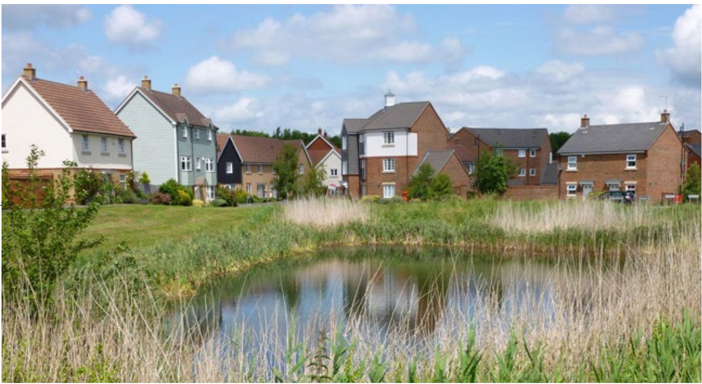
Surface water balancing area integrated into public open space design - with controlled outfall to existing surface water drain to Foxpound.
