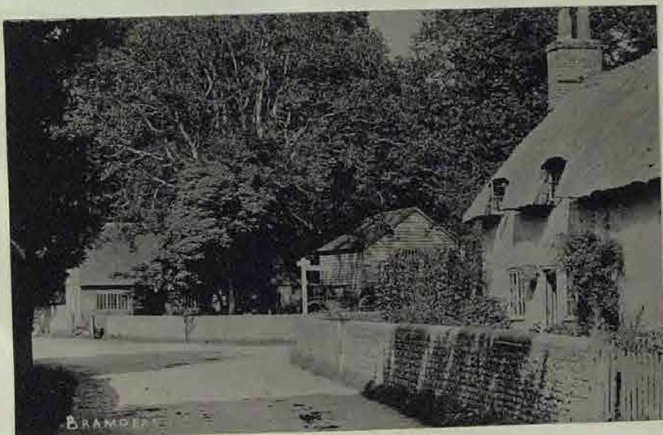
View of the old blacksmith's forge.
