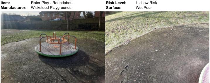
Finding: There is algae, silt or moss growth on the surface Action: Clean and treat appropriately resulting in slippery conditions
