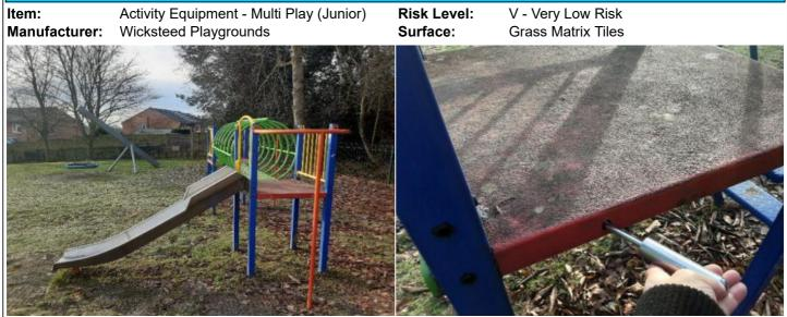
**Finding:** There is/are finger entrapment/s in the frame and the item fails to meet the requirements of BS EN 1176 Part 1 4.2.7.6 Entrapment of fingers
