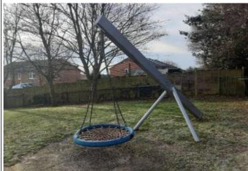
Finding: The incorrect seat design has been installed on this swing; there are unique designs for Type 1 and Type 3 swings that provide differing impact attenuating properties to the leading edges of the seat and/or has incorrectly aligned seat eye fixings which will lead to accelerated wear.
