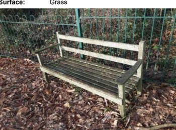
**Finding:** The bench/es is/are not securely fixed to the surface and there is some possibility of the item/s tipping or rolling over
