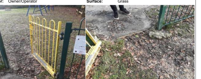
Finding: The area under the gate has eroded leaving uneven areas, or the concrete foundations exposed, resulting in trip hazards at the entrance/exit to the playground
