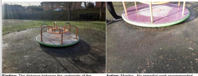
Finding: The distance between the underside of the roundabout platform and the playing surface is in excess of 110mm and contravenes the requirements of BS EN 1176 Part 5 which requires that the distance be maintained between 60mm-110mm - for the entire circumference of the roundabout
