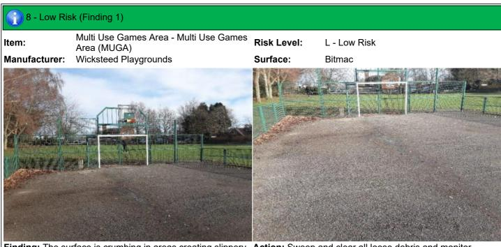
**Finding:** The surface is crumbing in areas creating slippery **Action:** Sweep and clear all loose debris and monitor conditions
