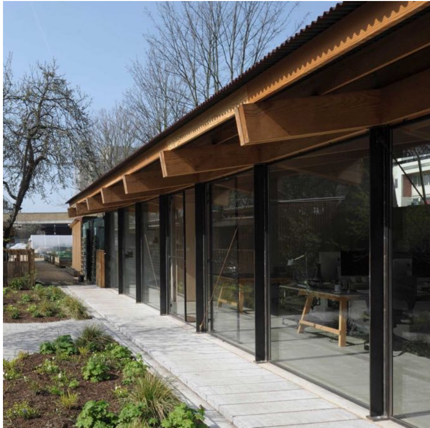
Roof overhang to control solar gain
