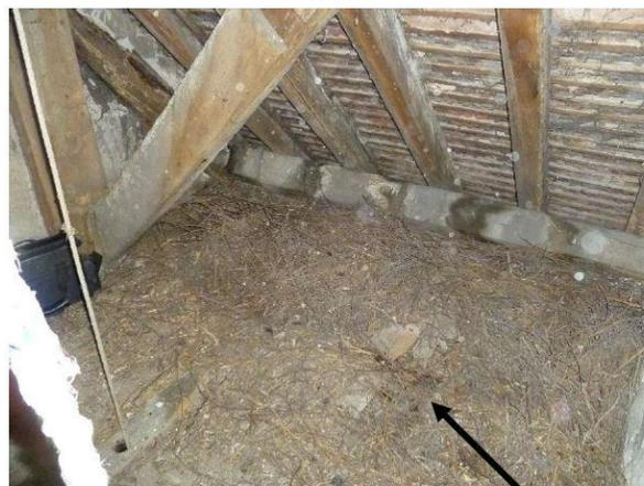
Fig. 4. Hole in the loft floor, largely concealed by detritus
