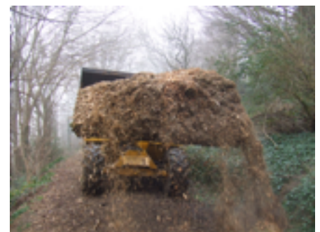
First Layer of Chippings on The Drive go down in March.
