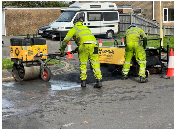
Much more environmentally friendly, lower carbon emissions, quicker and less disruptive to residents. It's not suitable for everywhere but offers a useful alternative to the traditional way by which patches of road that are breaking down are repaired and replaced.
