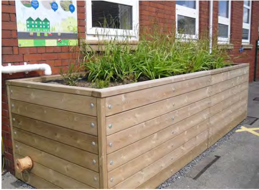
Downpipe fed garden planter
