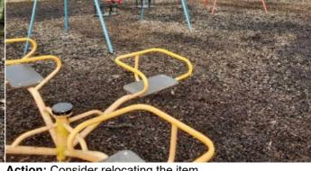
**Finding:** The falling space overlaps the free space between **Action:** Consider relocating the item the roundabout and the swings in contravention of the requirements of BS EN 1176:2017 Part 1
