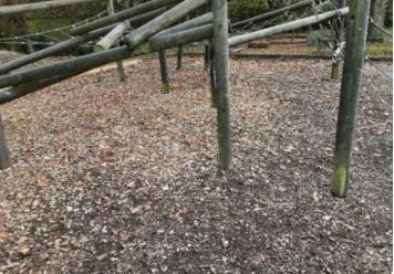
**Finding:** The depth of the loose fill surfacing is lower than the recommended depth specified in BS EN 1176 for a fall height over 2.0m. A minimum depth of 400mm is recommended (including an 100mm to allow for compaction and displacement as per BS EN 1176 Part 1 - Table 4)
