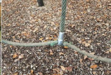
Finding: The ropes/nets are worn/damaged in places
