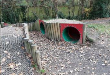
Finding: This design / configuration of tunnel mound is well Action: Monitor - No remedial work recommended established and has been successfully included in large quantities of playgrounds throughout the UK. Whilst the design does not fully meet the requirements of BS EN 1176 with regards to falls in excess of 600mm over the edge of the tunnel to the surface below, it has been risk assessed as fit for purpose and no changes are recommended to the design
