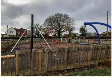
**Finding:** The loose fill safety surfacing has become compacted
