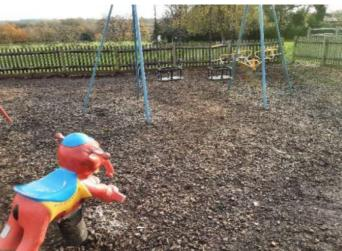
Finding: The falling space of the swings overlaps with an adjacent falling space in contravention of BS EN 1176 Part 2
