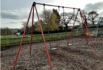
**Finding:** The chain links are worn in excess of 80% and require renewing
