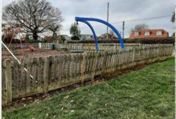
**Finding:** There are areas or parts of the timber on the fencing that have rotted
