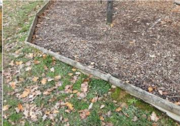
Finding: There is some evidence of rot in the timber edging Action: Monitor for any further deterioration and replace as
