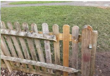
Finding: The fence is severely damaged in places
