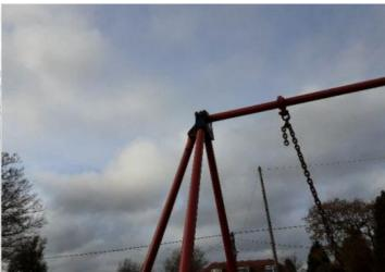
Finding: A number of fixing(s) have worked loose on the frame connections
