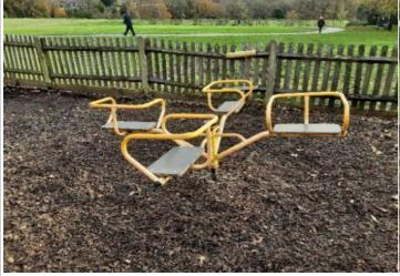
**Finding:** The fence forms a hard object within the falling space of the equipment and there is also insufficient surfacing provided in contravention of BS EN 1176 Part 1, 2000mm required, 1200mm provided
