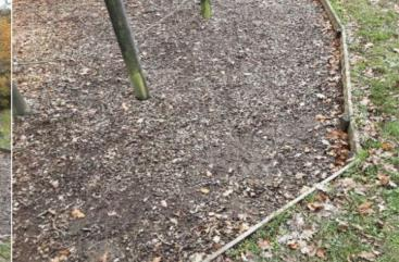
**Finding:** The loose fill safety surfacing has become compacted
