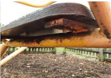
**Finding:** There is or are fixings missing on the underside of **Action:** Replace all missing fixings the seat
