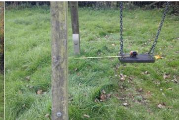
Finding: The seats are too close to the frame as defined in Action: Monitor - No remedial work recommended BS EN 1176 Part 2; this is a low risk failure and no remedial action is required
