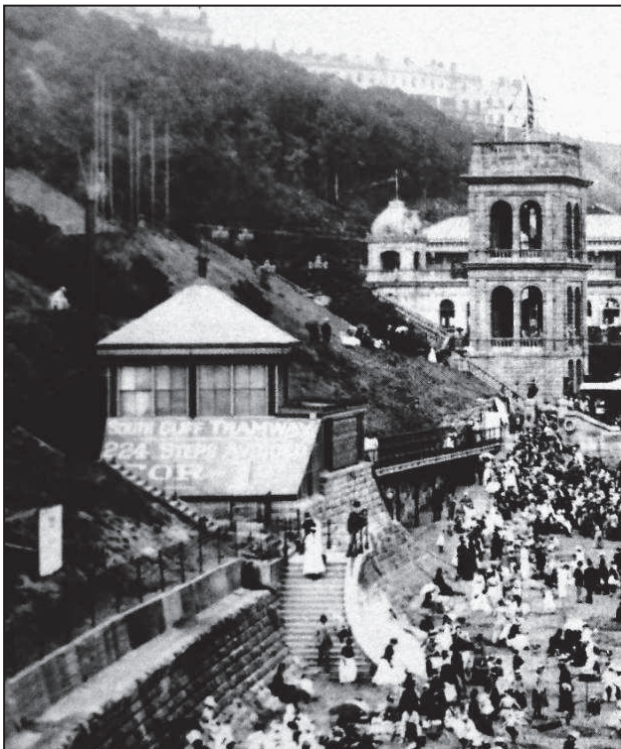
Plate 17. The Cliff Tramway shortly after construction and before widening of the promenade. The famous roof sign can be seen promising '224 steps avoided for 1d' as can the bridge from the spa (left). The winding path up the cliff can be seen on the south side, as can a small building over the tunnel beneath the tracks (below)
