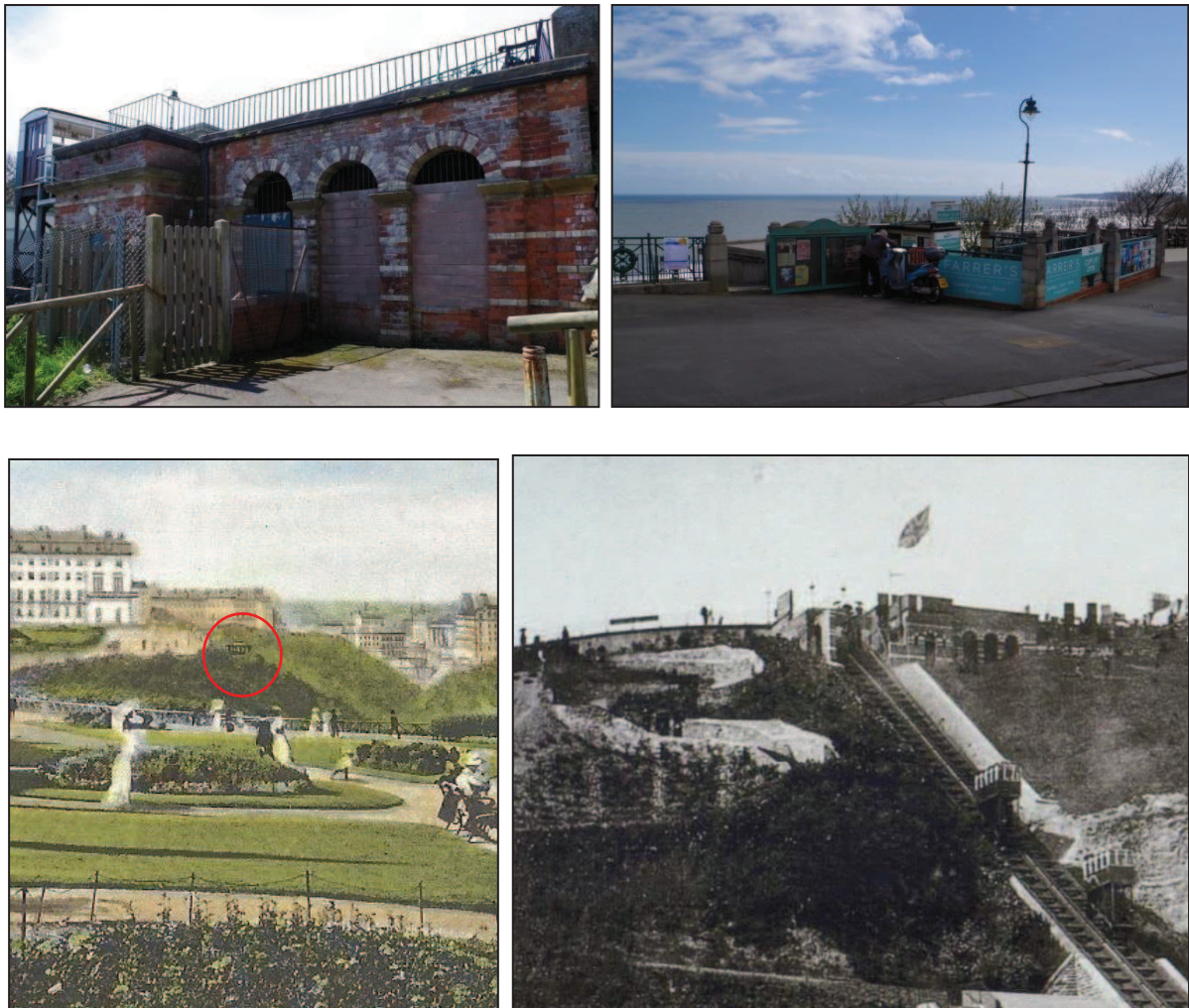
Plate 19. (top left) The top of the Cliff Railway appears to have originally consisted of the brick Italianate engine house for the hydraulic engine and water supply and a small cabin on the right/north of the track (bottom left). A larger cabin, similar in profile to that surviving at the promenade, seems to have been added by c.1900 (bottom left circled). Today the handsome and listed Italianate engine house is sadly neglected and fenced off. The current landscaping at the top of the railway is an early 20 th century scheme with failing precast concrete and overwhelmed by temporary poor advertising. Associated male and female toilets at the head on the steps on the south side are now closed.
