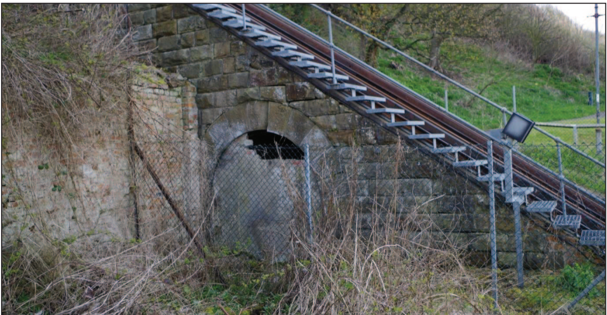
Plate 18. The pedestrian tunnel beneath the Cliff Railway of 1875. (Above) looking south as it goes beneath the steps parallel to the railway; (below) the finer quality stonework as the tunnel goes under the railway itself showing a slipped voussoir, single skin brick blocking and negative modern features of chain link fencing, metal steps and lighting. The area between the two tunnels was at one point covered by a small building (see plate 17).
