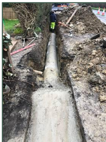
The main culvert successfully replaced in Paddock Wood
