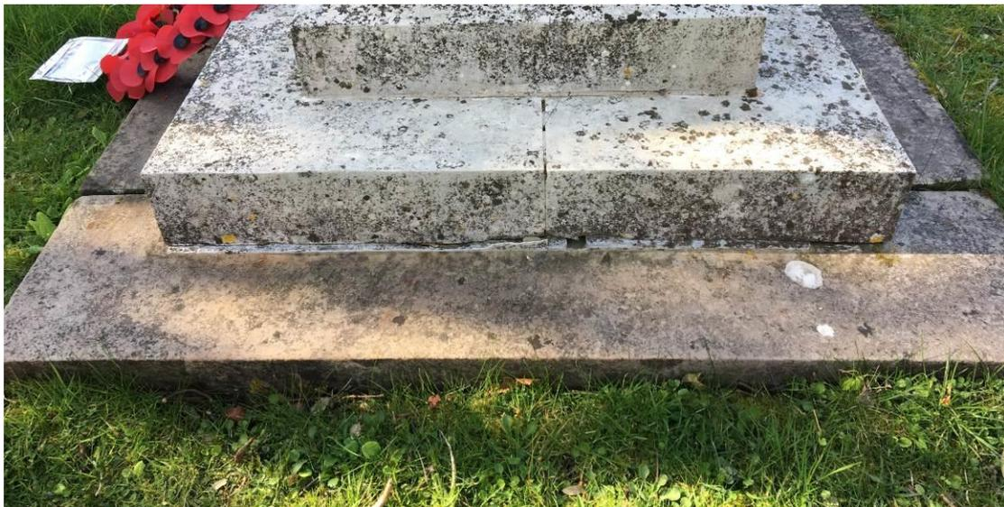
Fig.2 Detail of paving showing movement from tiered base.
