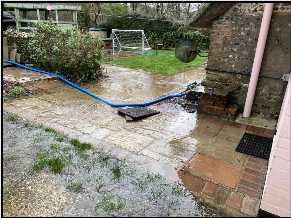
Fig. 2 Thatch End Foul Drain Propped Open to Take River Flooding
