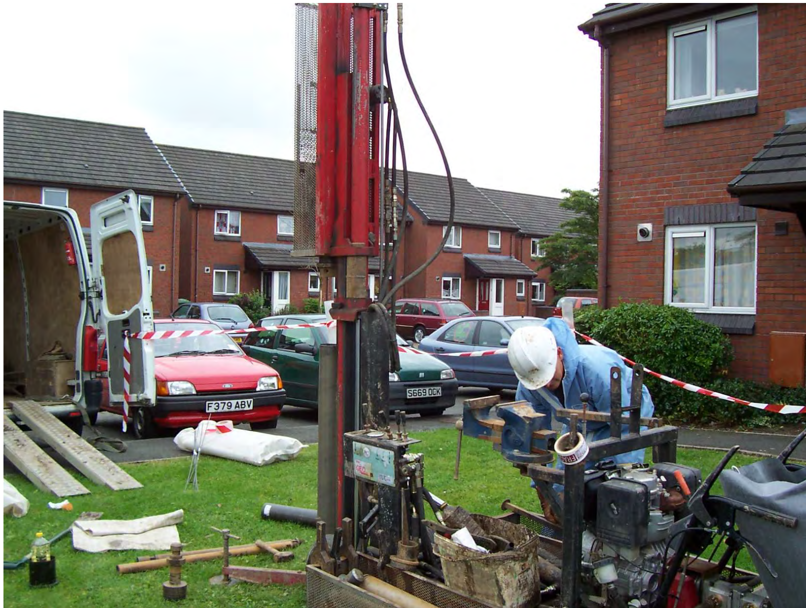
Figure 10 – Drilling boreholes in gardens
