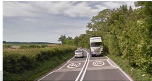
Provision of 40mph repeater roundels, coloured surfacing and tapered edge lines e.g. A31 Dorset
