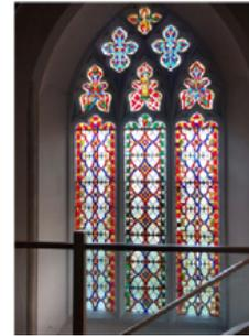
some glass is missing and the lead comes are bent. What's more, the whole light is distorted so the plan is to remove it, relead it and replace the missing pieces with newly painted quarries to match. Fortunately, the Friends of Kent Churches
