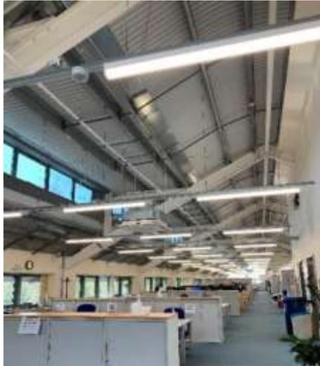
KCC have switched the lighting at the Highways Henwood offices / depot in Ashford to light emitting diodes (LEDs). 109 lights were replaced with LEDs including in the office, car park, storage building, flood lights and streetlights. Five KCC libraries have also moved to LED lighting. The total energy savings for these projects is estimated as over £96,000 per year (this figure was calculated before the energy price increases experienced this year).
