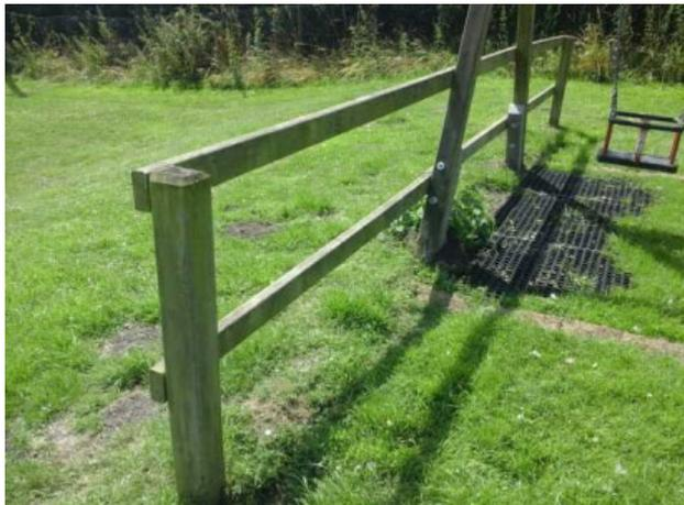
**Finding:** The posts on the swing barrier are slightly loose in the ground
