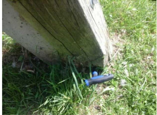
**Finding:** There are areas or parts of the posts on the structure that have rotted
