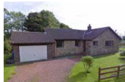
Existing bungalow development
