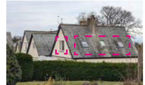
Varied roof line & roof lights
