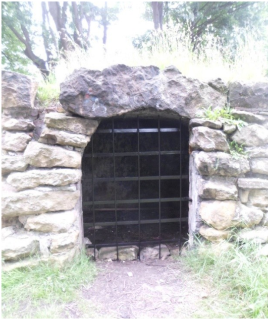
The new door on the Ice House
