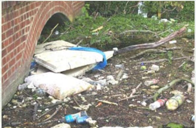
Photo 10: Restricted flows through a partially blocked culvert can increase the risk of flooding.
