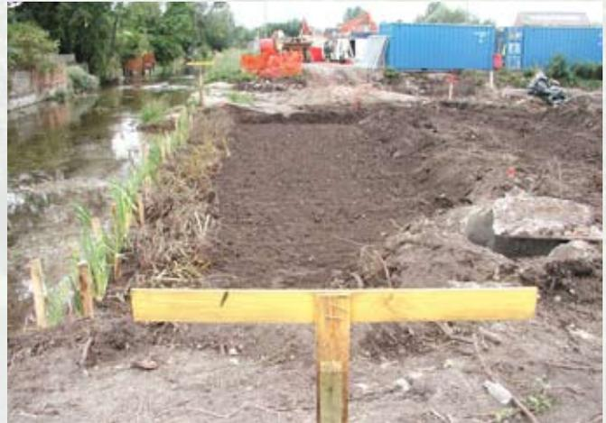
Photo 23: New wetland habitat under construction during redevelopment beside the River Anton at Anton Mill Road. This new habitat will replace tarmac and concrete, which previously extended to the river's edge
