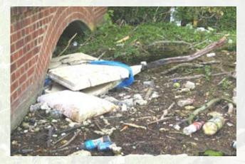
Photo 10: Restricted flows through a partially blocked culvert can increase the risk of flooding.
