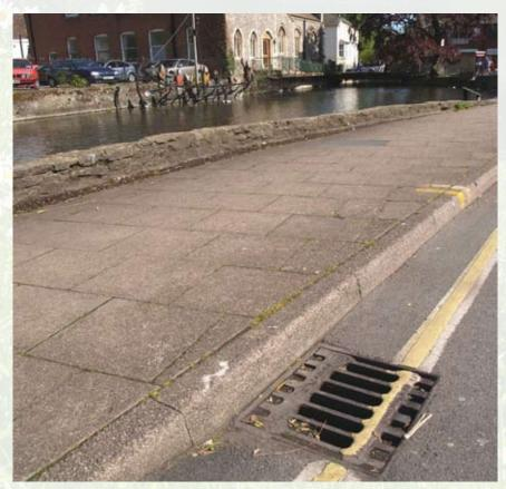
Photo 13: Surface drainage, e.g. from roads and other paved areas, frequently carries a high sediment load and discharges directly into the river.
