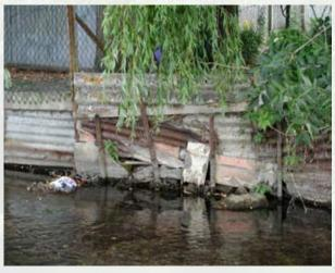
Photo 5: Make-shift revetment constructed from corrugated iron. Revetment like this offers no habitat value and, if washed out, could block downstream culverts and cause flooding.
