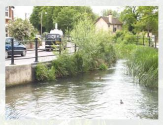
Photo 22: Wetland vegetation is encouraged to provide habitat and to screen the steel sheet piling, which forms the river bank in Bishopstoke
