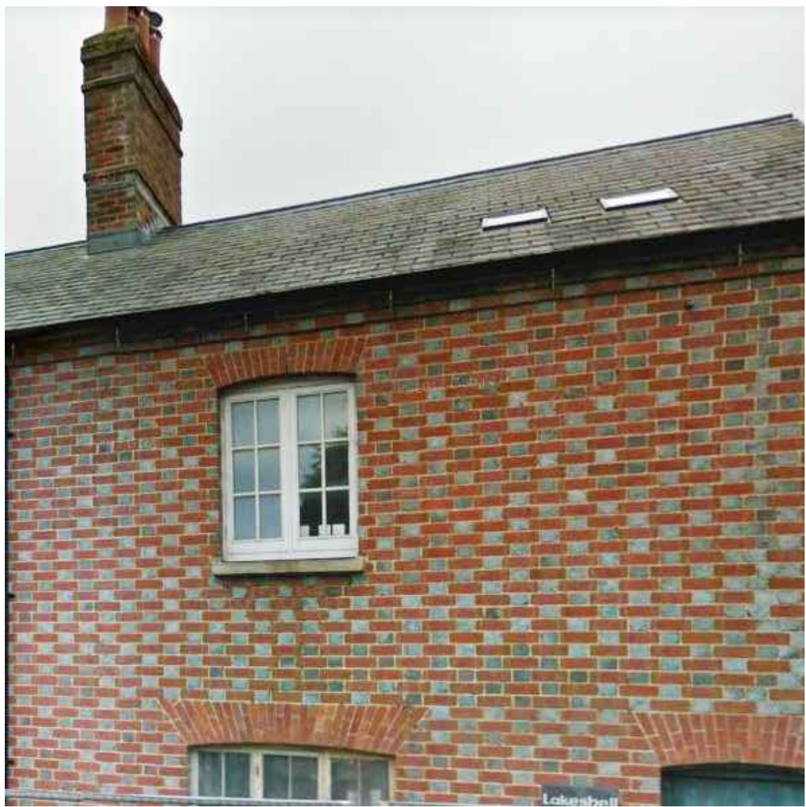
FLEMISH BOND BRICKWORK
