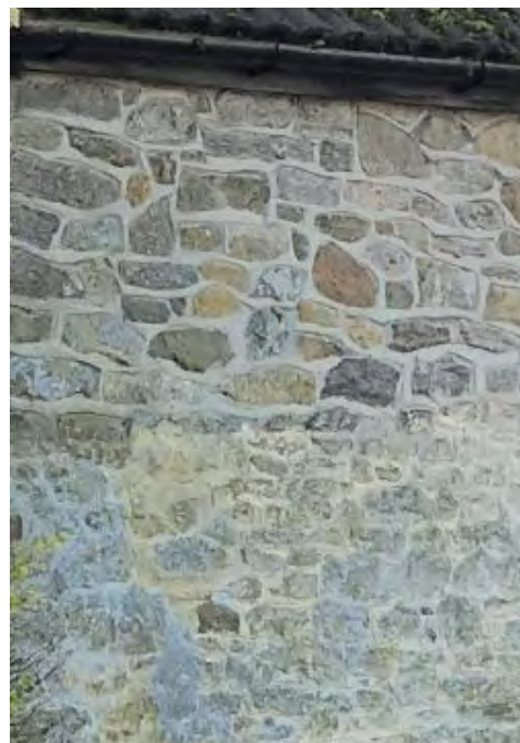
Fig 23. Pottinger Cottage 1790. First floor level stonework replaces a partial collapse caused by the removal of thatch. Limewash traces.
