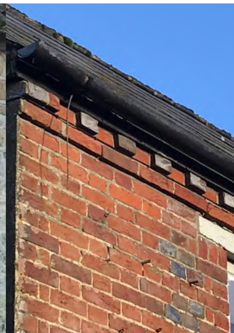
Fig 24. Crowdy's, 1801. Flemish bond variant brickwork with dentilation with vitrified headers below eaves.
