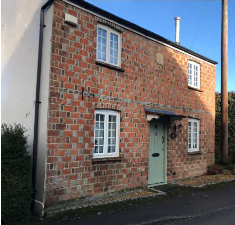
Berry Hill Cottage, 'AD 1854' on date plaque. Of brick in an unusual rat-trap and header bond.
