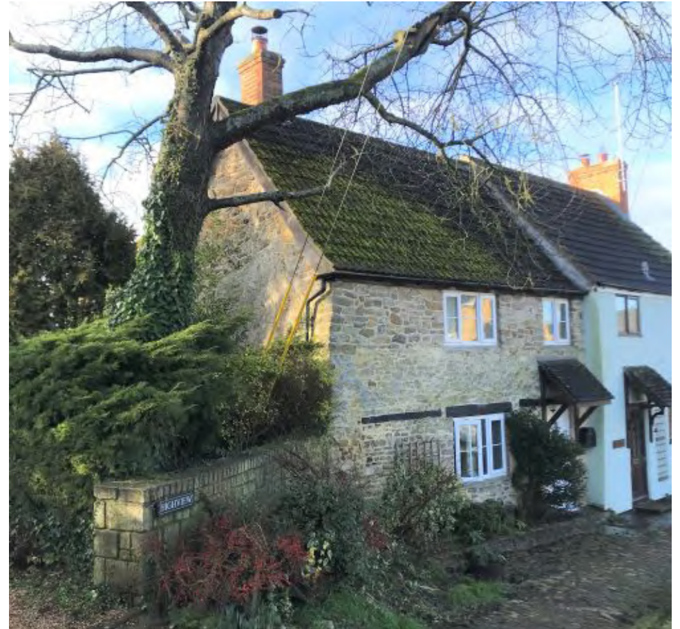
Pottinger Cottage, 1790 Irregularly coursed stone rubble with irregular stone quoins, some butter-pointing. More regular coursing at first floor level replaces a part-collapse when the earlier thatch was removed. Wooden lintels over four three- and two-light casement windows (another blocked). Brick chimney stack through ridge within house, thus several features earlier than date given.
