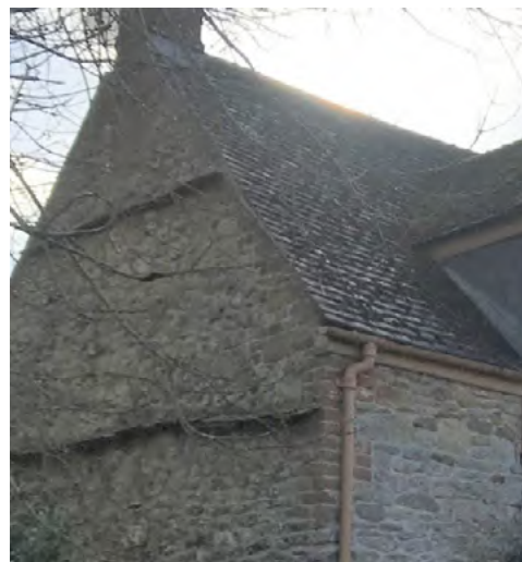
Fig 27. Hillside c 1801. Brick quoins from first-floor level where house extended upward. Stone slate dripstones in three courses to the north-facing gable end below chimney.
