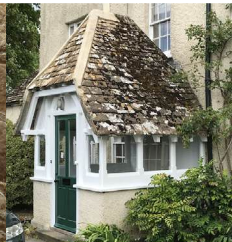
Fig 22. Glebe House 1790. Timber and rendered half-hipped porch with stone tiles.
