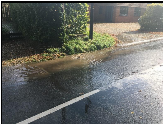
Fig 4 showing a blocked drain on the B3046.
