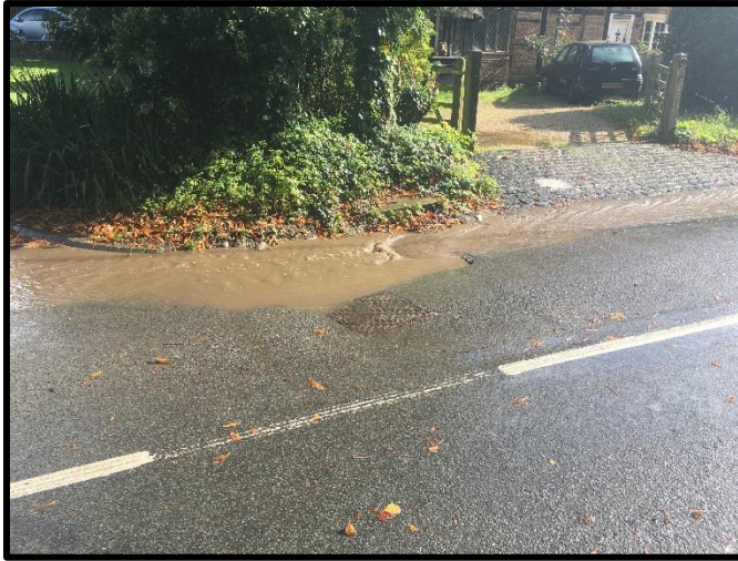
Fig 5 showing a blocked drain on the B3046.
