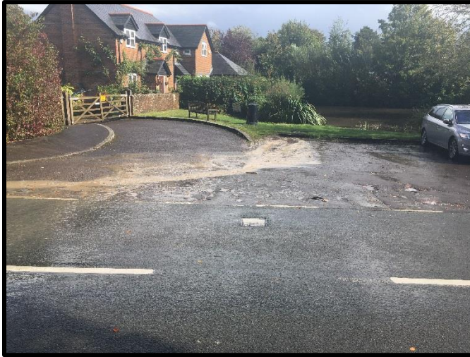
Fig 10 Showing the flow from Woods Lane eventually entering a drain approx. 3 metres from the pond.
