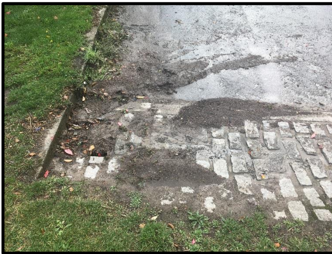
Fig 11 Showing the silted up drain into which the run off from Woods Lane enters.
