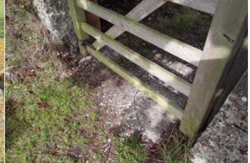
Finding: The area under the gate has eroded leaving uneven areas, or the concrete foundations exposed, resulting in trip hazards at the entrance/exit to the playground
