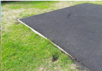
**Finding:** There are trip hazards at the edges of the wet pour **Action:** Reinstate surrounding surface levels to remove the surfacing trip points
