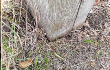
**Action:** Monitor for any deterioration (rot) and replace as required
