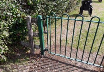
Action: Take corrective action to ensure that the gate closes in 4-8 seconds
