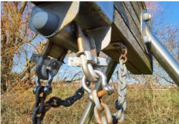
Finding: The pivot mechanism fixings are corroded
