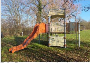
**Finding:** The tree canopy overhangs the equipment and is less than 2.0m away
