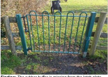
Finding: The rubber buffer is missing from the latch plate
