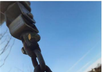
**Finding:** A number of fixing(s) appear to have worked loose **Action:** No further action required - but they have been welded
