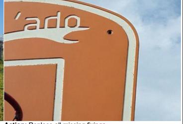
**Finding:** There is or are fixings missing on the backboard
