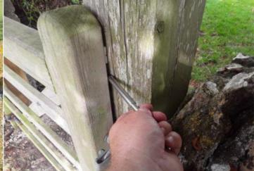
**Finding:** There are openings that are less than 12mm that could trap or crush fingers
