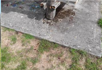
**Finding:** There are trip hazards at the edges of the concrete **Action:** Reinstate surrounding surface levels to remove the pad trip points
