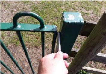
**Action:** Where possible a 12mm gap should be maintained on both sides or between the gate leaves
