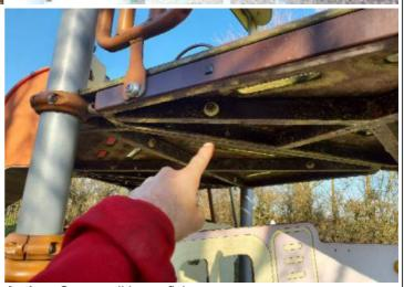
**Finding:** A number of fixing(s) have worked loose beneath **Action:** Secure all loose fixings the platforms
