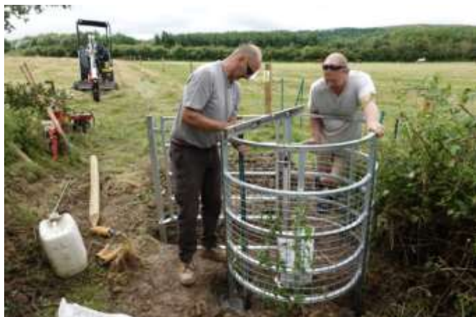
Mario and Andi, of Pepler Fine Fencing Ltd, at work on kissing gates 8/9:
