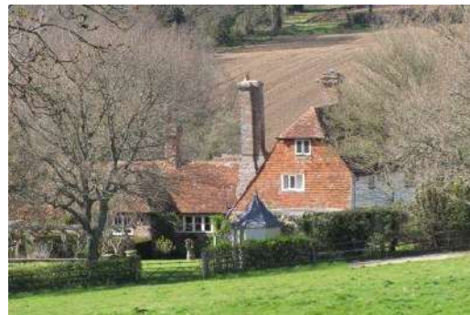
Combe Farmhouse (south side)
