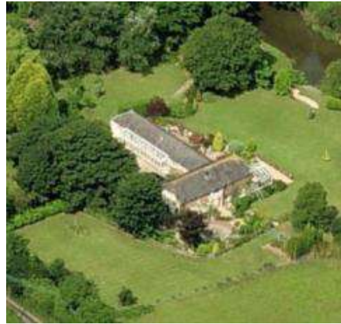
Whitehaven (former Parish Workhouse)
