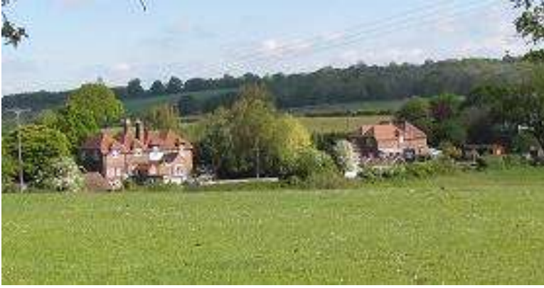
Former Brickyard Cottages (rear)
