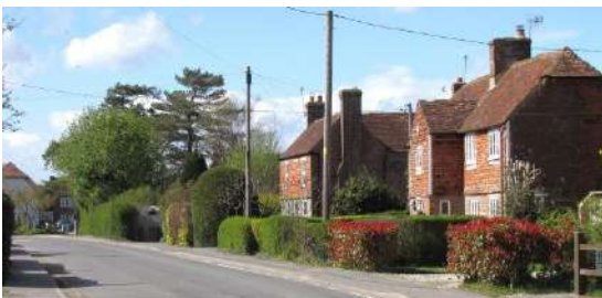
1-3 Fir Tree Cottages & Fir Tree House
