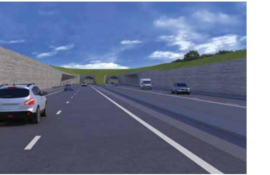
Figure 5.27: Driver's view of western tunnel entrance - vertical retaining walls option
