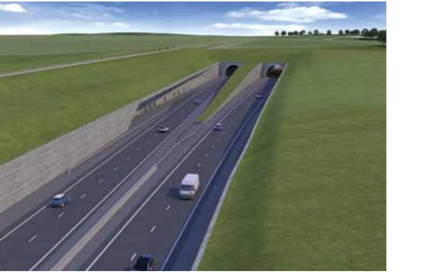
Figure 5.26: Western tunnel entrance - vertical retaining walls option
