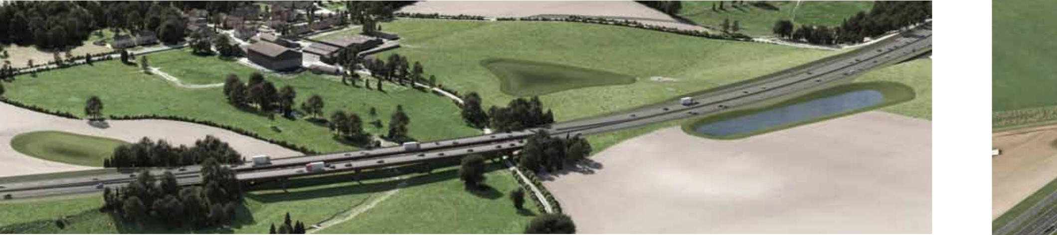
Figure 5.12: Road drainage infiltration areas either side of the River Till
