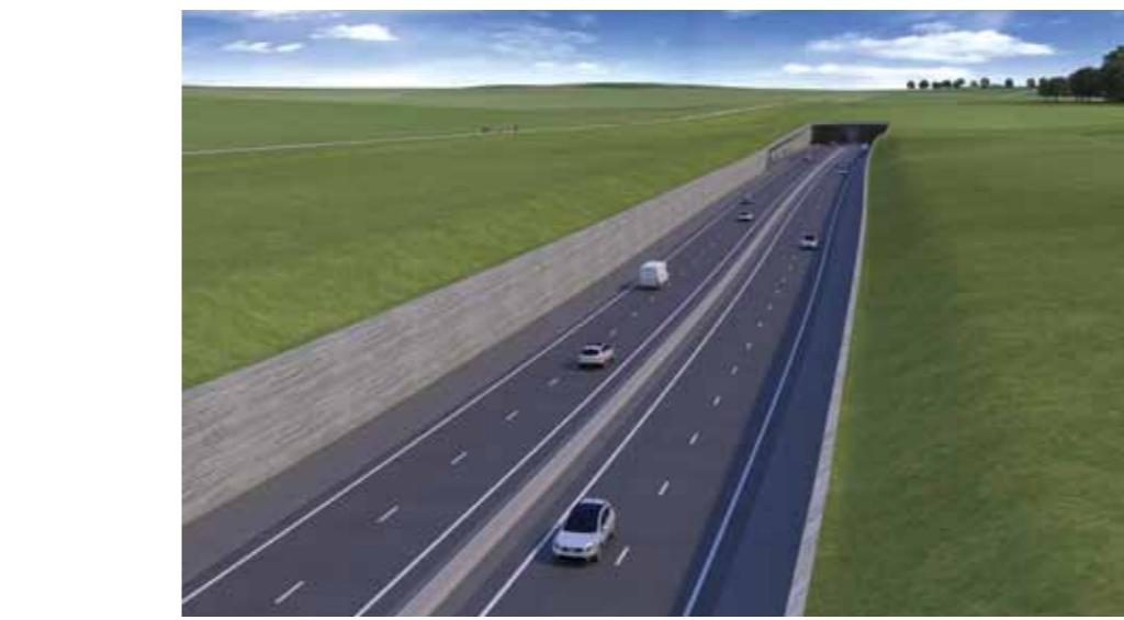
Figure 5.22: Approach option with vertical retaining walls
