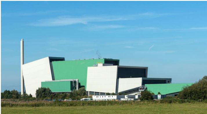
Javelin Park Incinerator
