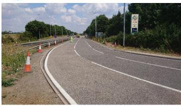
A5 resurfacing and new anti-skid laying on the approach to the roundabout
