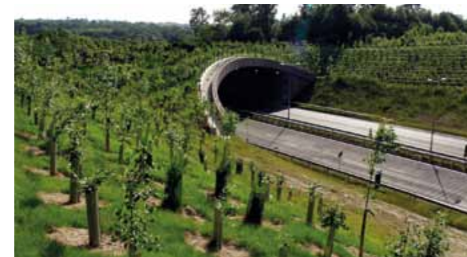
An example of a green bridge
