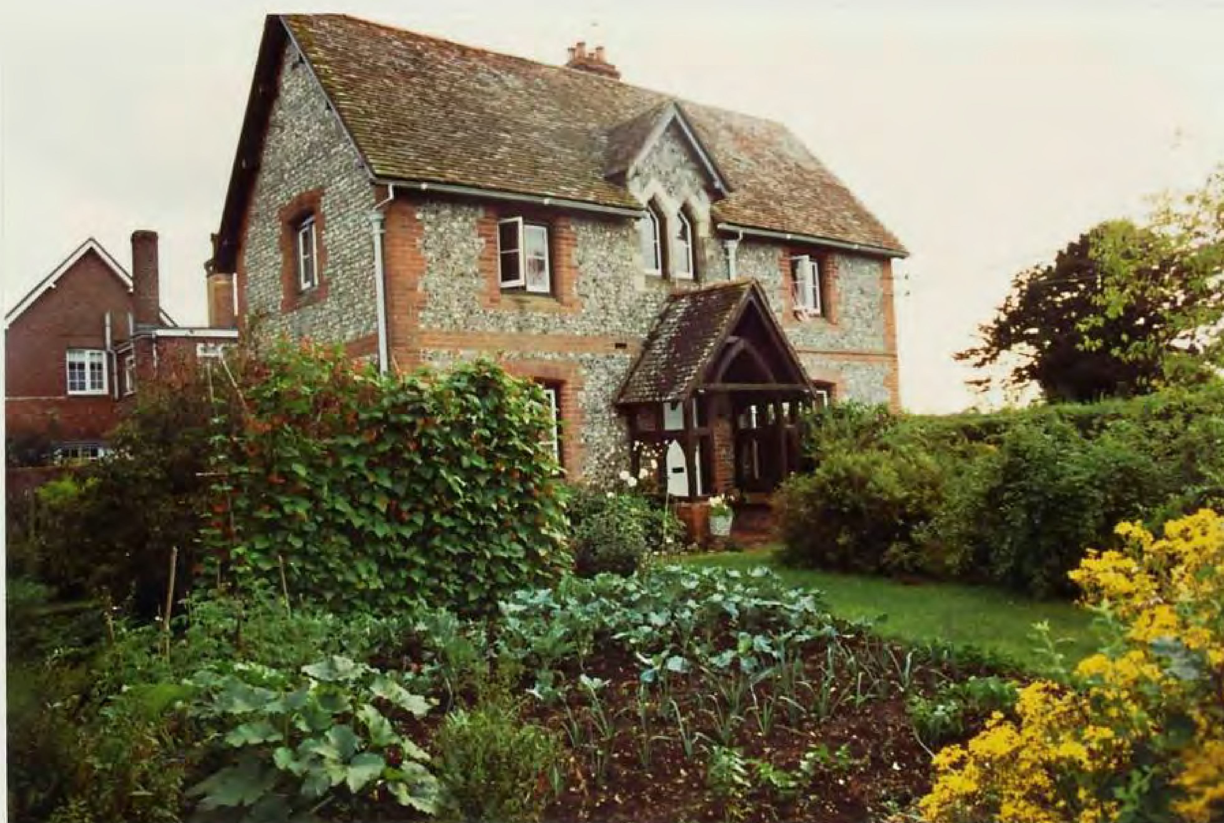
1 Church Cottages, Kilmeston
