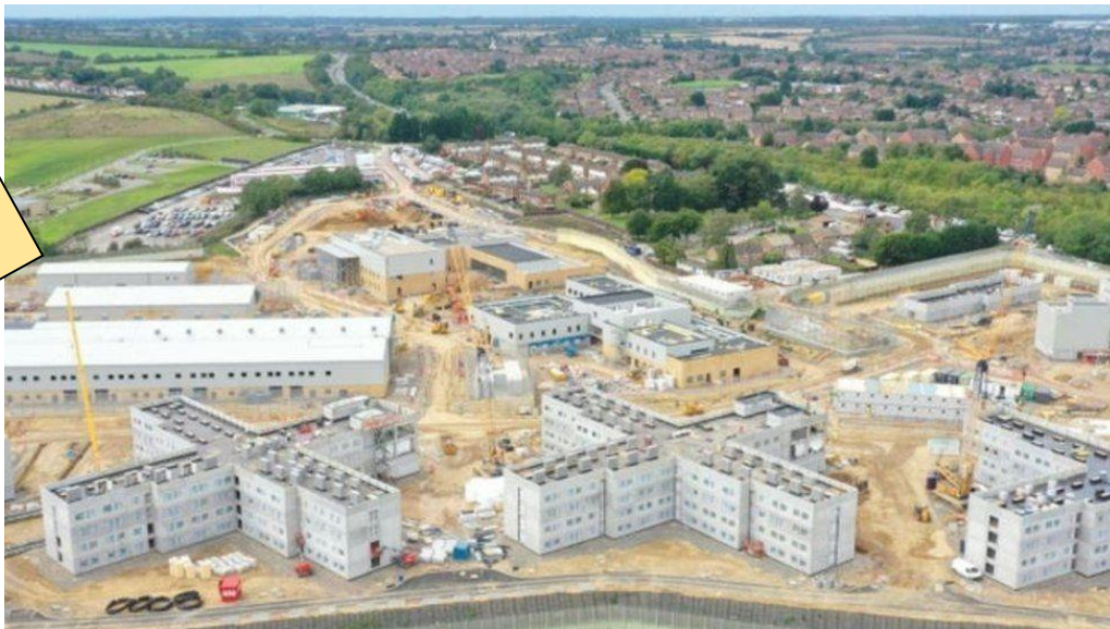
The new prison being built at Wellingborough
