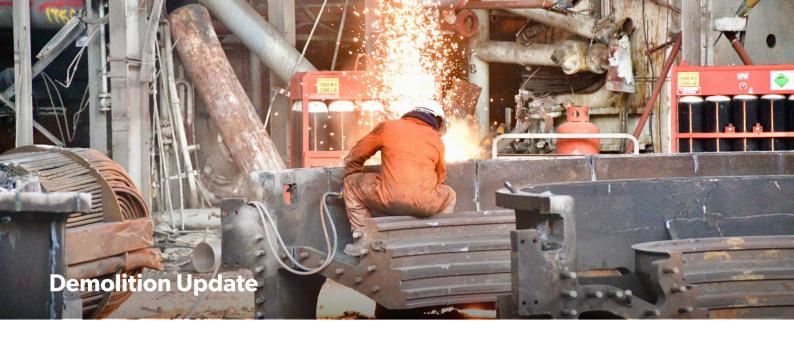
Our demolition programme is progressing well, with the scheme on-time and on-budget. The team has now entered into the turbine hall and begun the removal and scrap of old equipment, as can be seen from the photos above and opposite courtesy of John Bray at the BBC.
