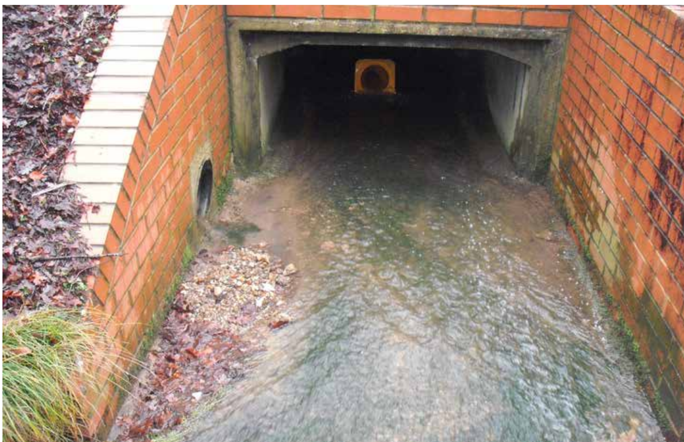
Detritus in the culvert leading from Ewshot Lane under Redfields Lane at 11am 4 Jan 2014
