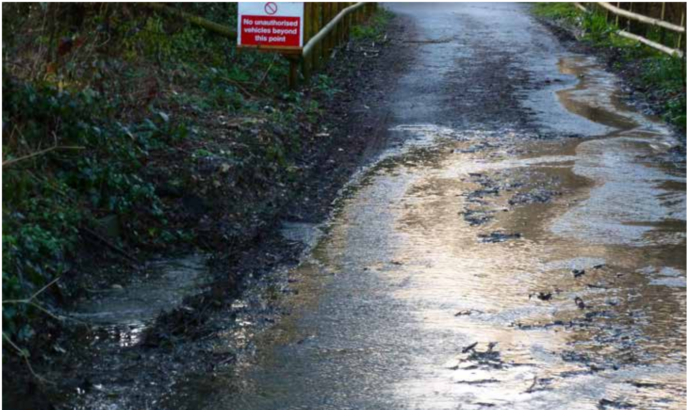
Showing the route of water from the roadway into the main stream (after the main flow had subsided)
