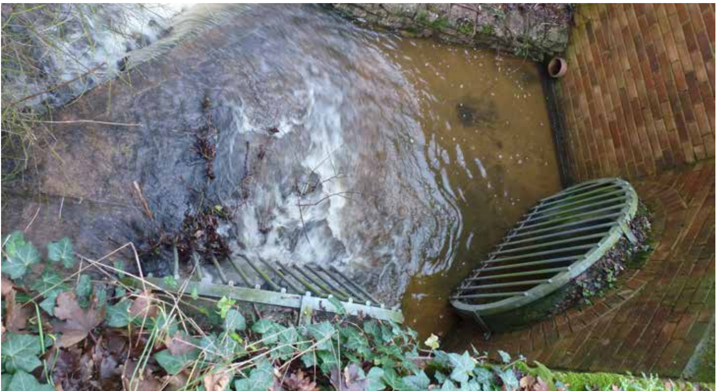
Culvert (R) into Brandon Road ditch appears blocked upstream 2:30pm 6 Jan 2014
