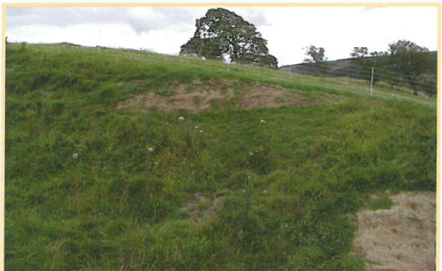
Turf stack repair two months later
