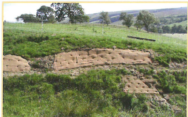
Turf stack repair on completion
