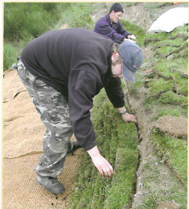
Turf stack repair being constructed.
