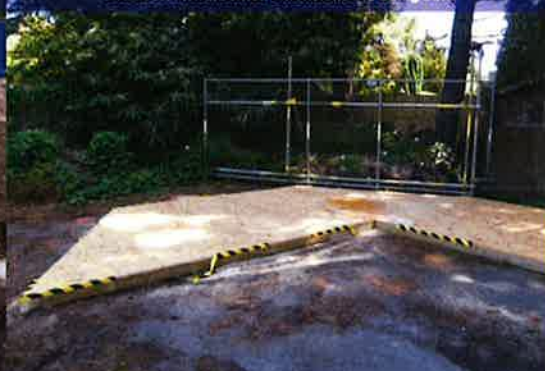
Image 4: Existing surfacing can be used as ground protection and reinstated near the end of development
