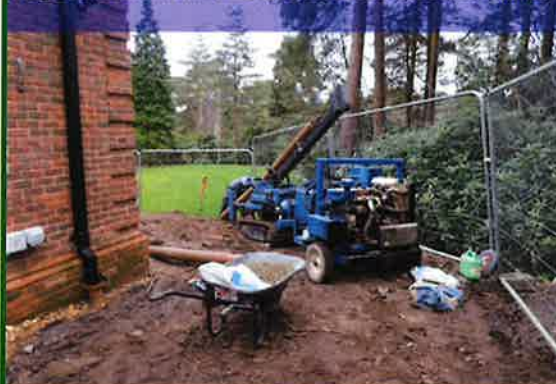
Image 3: All operations must be carried out on the development side of the tree
