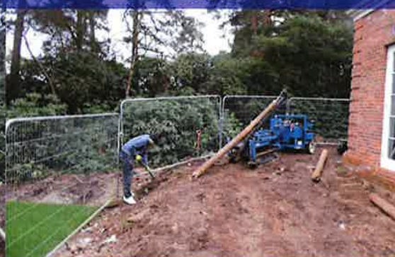
Image 4: Once the pile has been installed in the ground, the foundation can be cast to avoid any excavations
