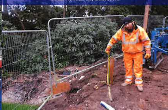
Image 4: Once the pile has been installed in the ground, the foundation can be cast to avoid any excavations
