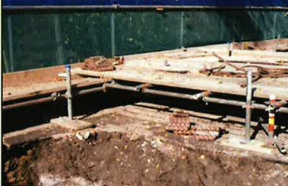
Image 5: Concrete slabs formed on site can make useful ground protection for heavy construction machinery
