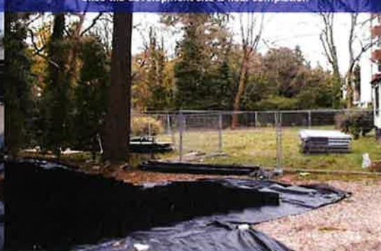
Image 6: Geocell can be used as temporary ground protection and lifted once the development site is near completion
