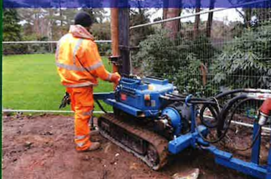
Image 3: All operations must be carried out on the development side of the tree
