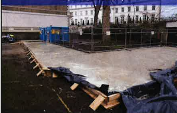
Image 5: Concrete slabs formed on site can make useful ground protection for heavy construction machinery
