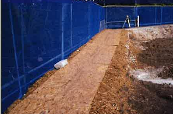
Image 3: Ground protection can be erected on scaffold platforms to prevent foot traffic from compacting tree roots
